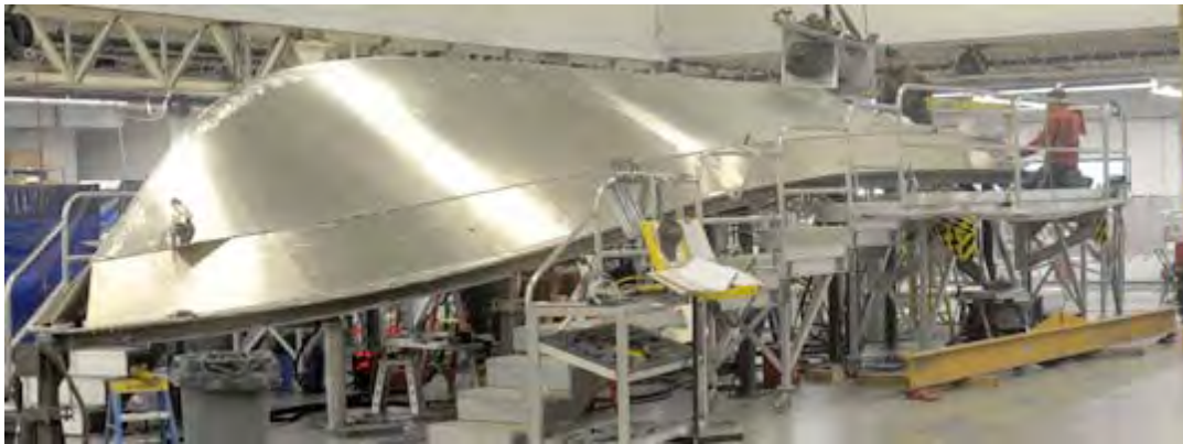
The hull off an RB-M is assembled on a jig. Photo by PA2 Dan Bender
