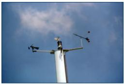
Despite the installation of a fuzzy lightning" the bolt ignored the taller VHF antenna and hit the dissipater.
